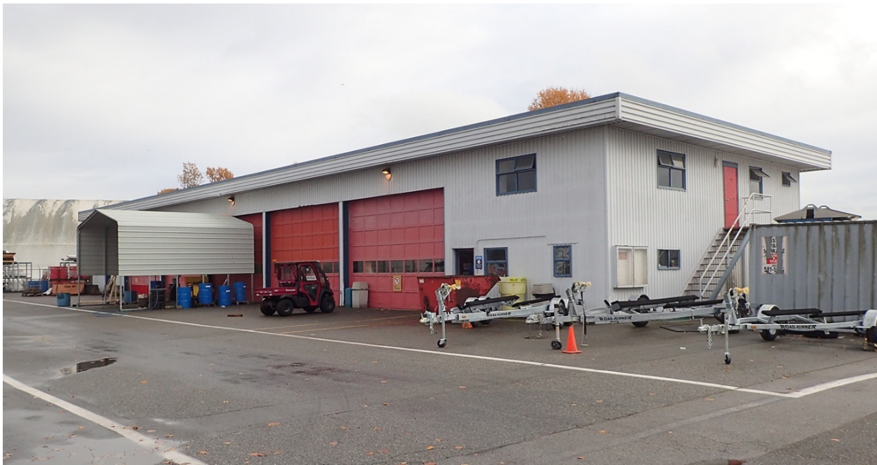
FIGURE B-7: RESCUE BOAT SHOP
