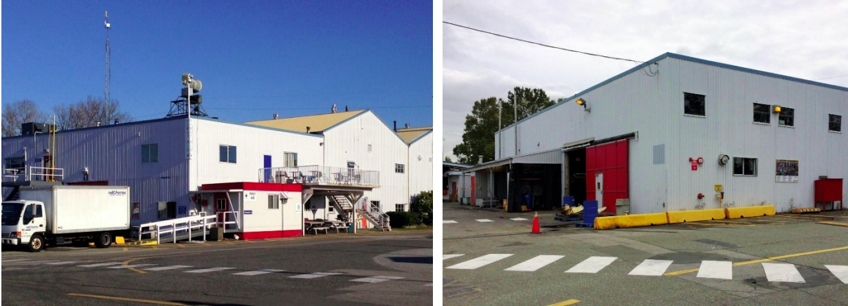
FIGURE B-3: MACHINE SHOP (LEFT) AND HEAVY SHOP (RIGHT)
